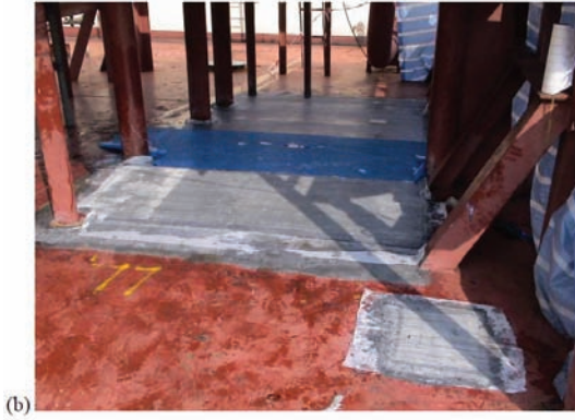
Figure 1 Composite patch repair of the corroded deck floor of the FSO ABU Cluster ( (a) shows the deck before the repair), (b) shows the deck after the repair)
